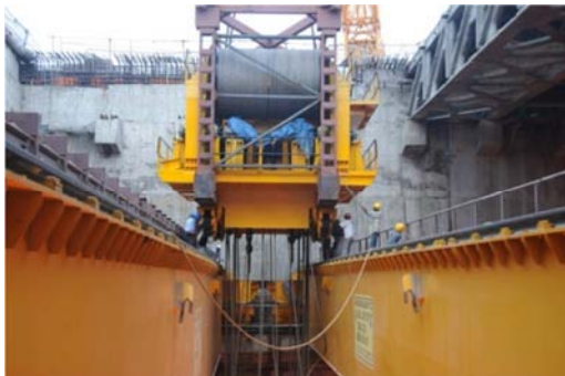
Figure 6. Trolley assembly being placed with the hooks on the bridge girder rails.
