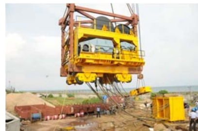
Figure 5. Trolley assembly being lifted with the hooks.
