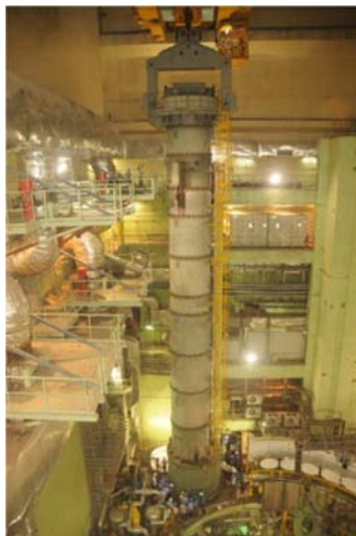
Figure 11. PI Flask (230 tons) lifted inside RCB.
